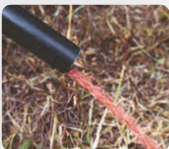
Application of granules
